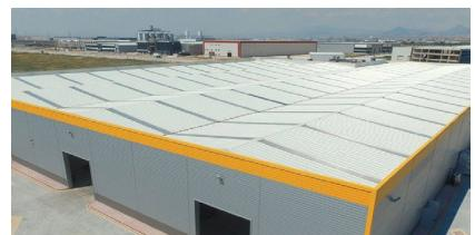
**5 HADVELİ ÇATI PANELİ / 5-PITCH ROOF PANEL / PANNEAU DE TOIT A 5 NERVURES**
